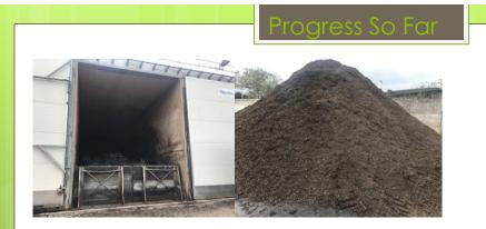
The process would involve reception of waste in a sealed negative pressure building, shredding and mixing of waste, then storage of waste in an enclosed composting tunnel before being transferred to an outdoor aerated static pile composting facility for stabilisation/maturation and then screening. Any unsuitable material would be sent off site to be re-processed into a biomass fuel for energy and/or heat recovery.
