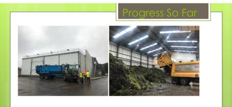
The application site area is approximately 1.2 hectares. The application proposes to develop an organic waste in vessel composting (IVC) facility to manage up to 75,000 tonnes per annum of compostable municipal green and food waste. This would involve a mixture of invessel composting (IVC) within a purpose built building, and external aerated maturation using a system of forced aeration static windrows.
